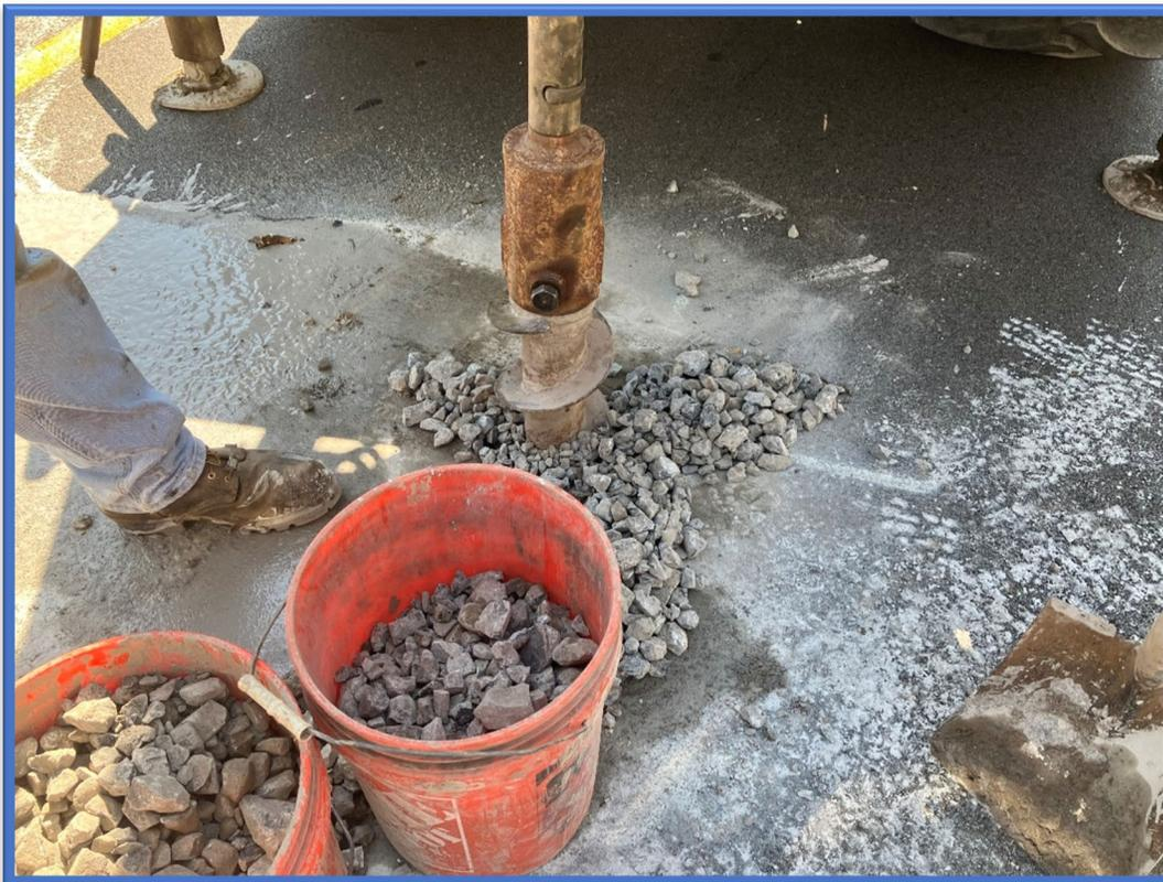
Photo 4 - Engineered fill / blast rock present beneath the asphalt/concrete roadway surface at FH-X-27e.
