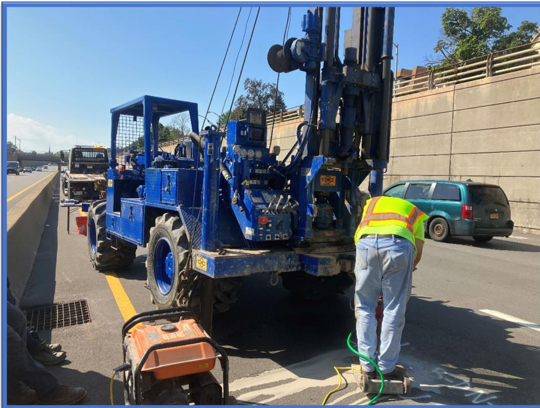
Photo 3 - CME coring through the asphalt/concrete roadway layer prior to utilizing the hollow-stem drilling augers and split-spoon sampler to retrieve the subsurface soils.
