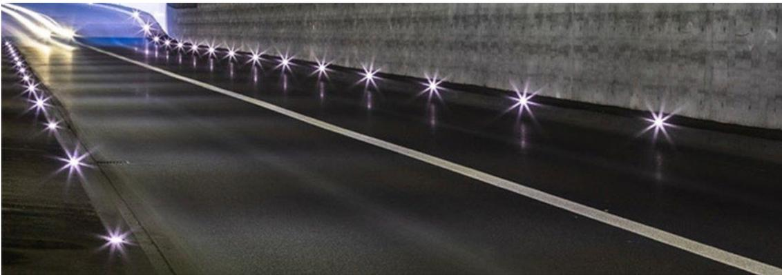
Figure 5: LED Floor Guidance Lights
