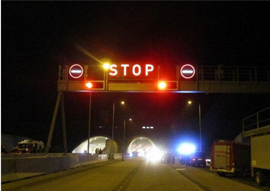
Figure 9: Traffic Signals at Tunnel Portal
