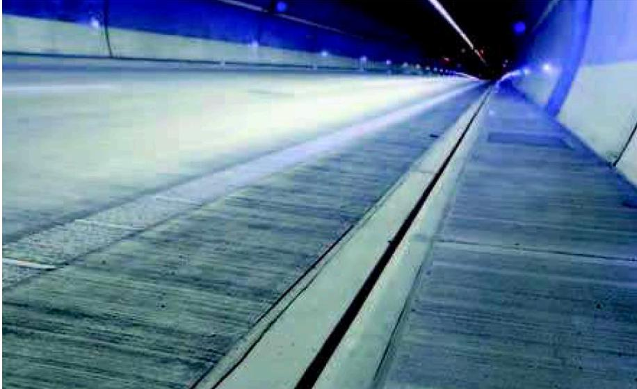
Figure 13 Slotted Channel for Drainage
