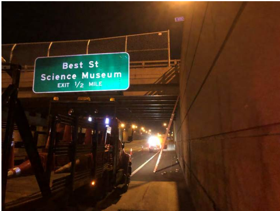
Photo 3 – View looking south at BIN 1022630 (E. Utica Street over Kensington Expressway (NY Route 33)). MPT was necessary in order to inspect the underside of the bridge.
